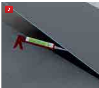
... apply building boards, seal ...
