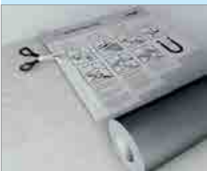
Cut membrane to size ...
