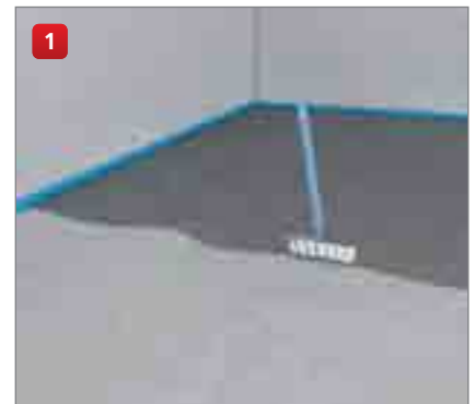
1 Clean and prime ...
