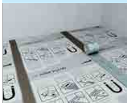
... seal joints if necessary.
