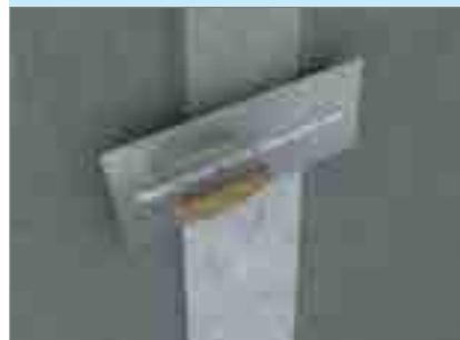
... level, abrade, coat, done!
