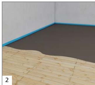
2 Apply tile adhesive to the wooden substrate.
