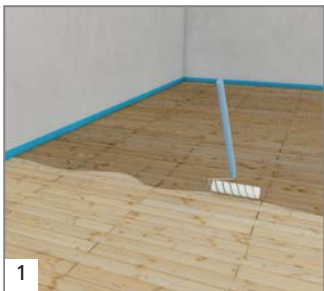
1 Prepare wooden floor with primer.
